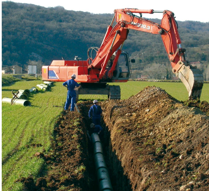
FIGURE 7.3: Pose de canalisation [7]
