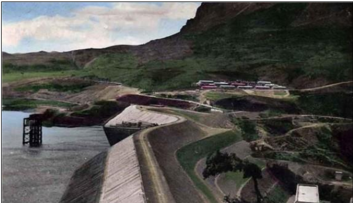
Figure III.2 La digue du barrage de MAHOUANE (Source: ALGERIE PRESSE SERVICE, 2019)
