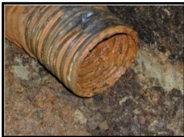
Figure VII.2:Le colmatage des drains
