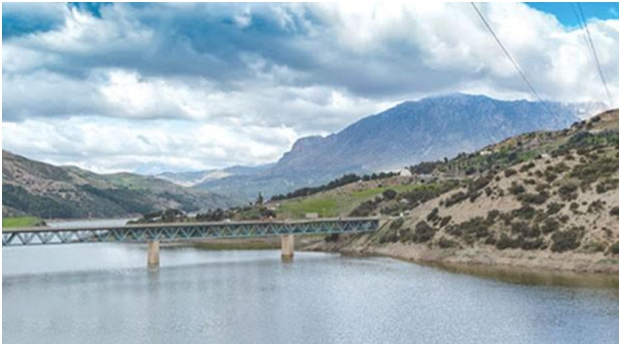
Figure III. 3: Barrage de MAHOUANE. (source :ONID)
