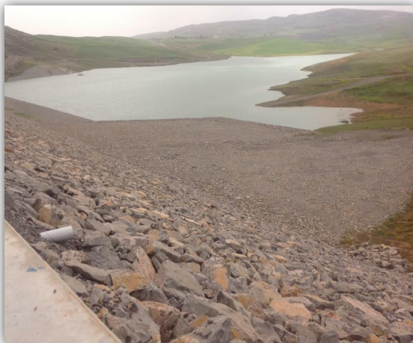
Figure III. 1: Barrage de MAHOUANE.
